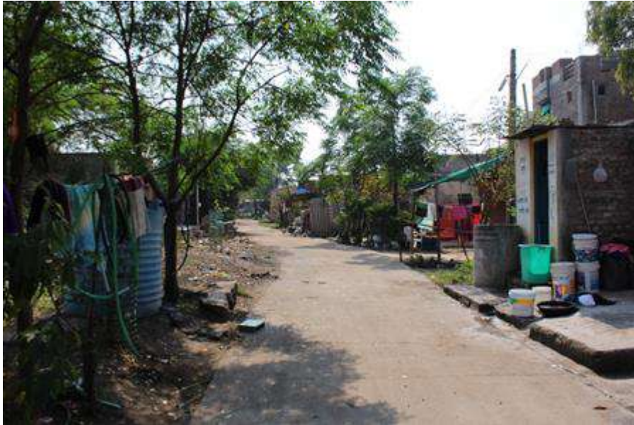
Image 7.5: Internal Concrete road
