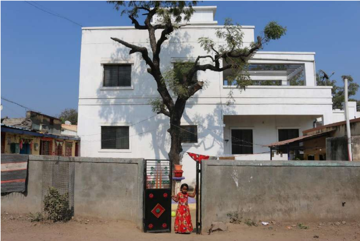
Image 5.6: RCC House in Guha Village (Source: Author)
