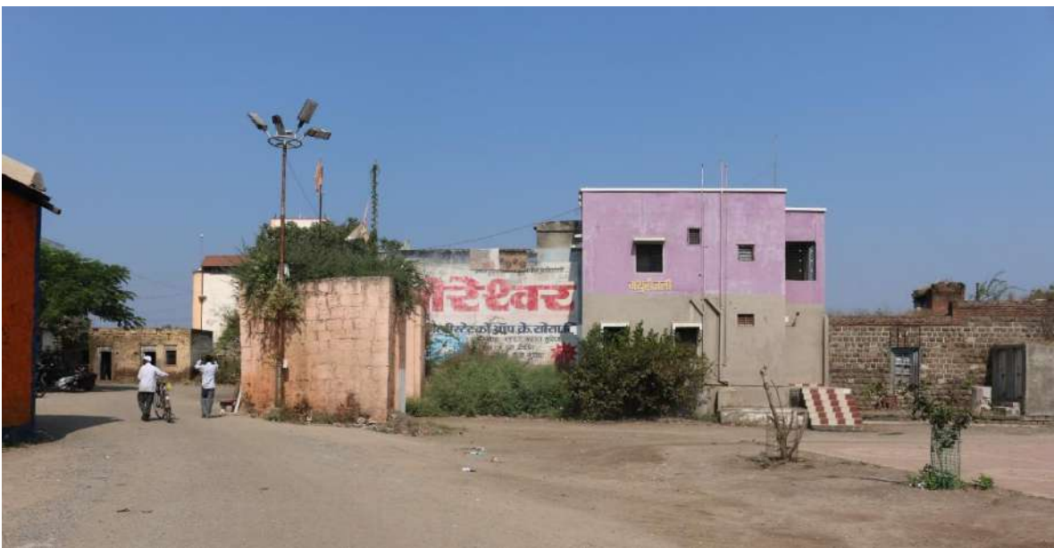
Image 5.7: RCC Structures in Guha Village (Source: Author)
