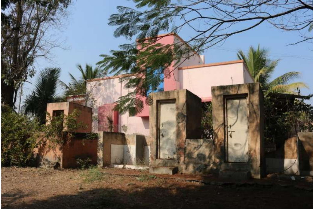
Image 5.8: RCC House in Guha Village (Source: Author)
