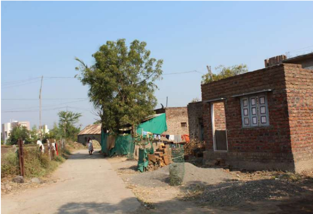
Image 5.2: Brick House in Guha Village (Source: Author)
