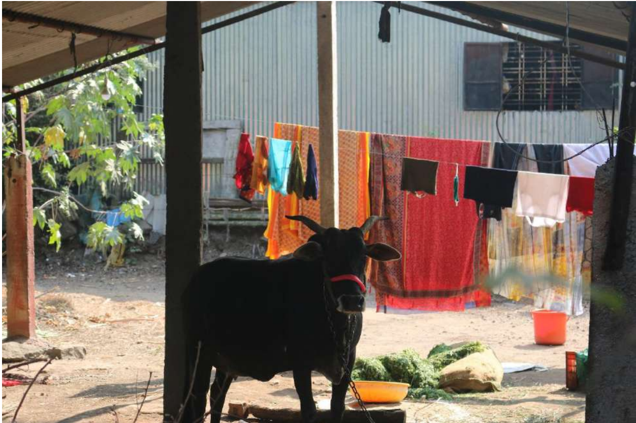
Image 5.10: Metal roof Cattle Shed
