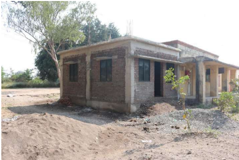
Image 5.9: Under Construction Houses in Guha Village (Source: Author)
