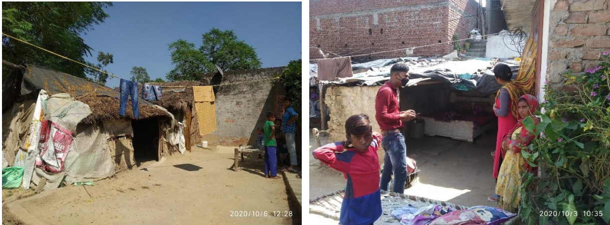
Figure 35 Dilapidated housing condition of poor rural people, Source- IITR survey team
