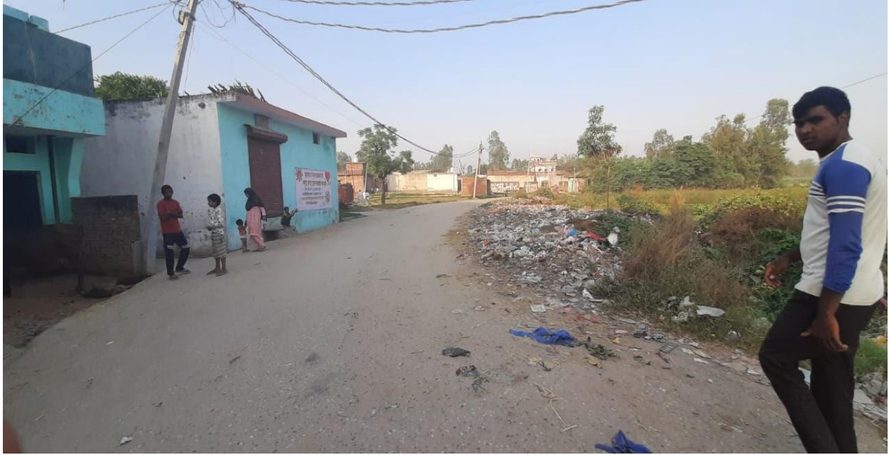
Figure 42 Cement concrete (CC) roads to the agricultural land
