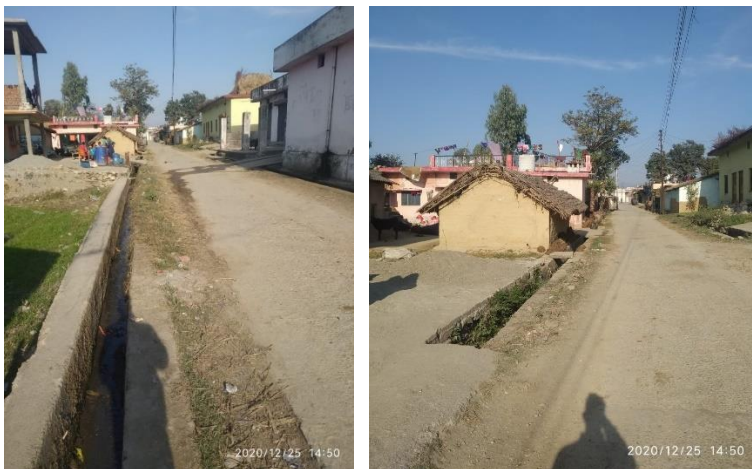
Figure 66 Open and semi open surface drains are present in the village in Chharba.
