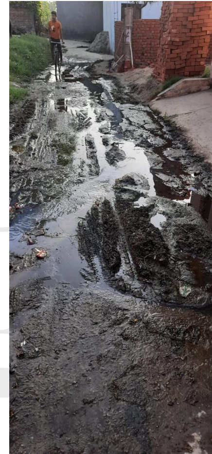
Wastewater flowing over access roads
