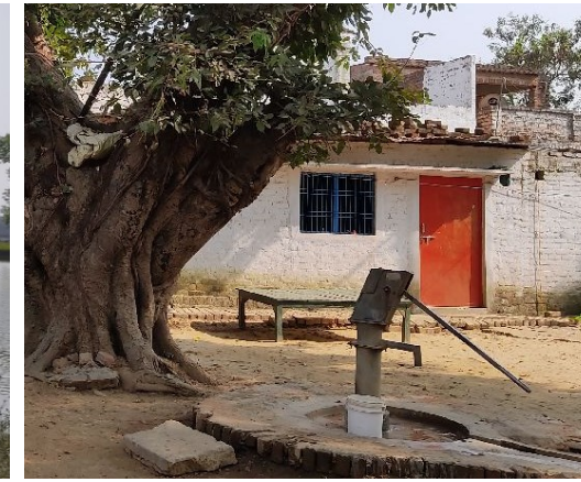
Hand pump outside HHs
