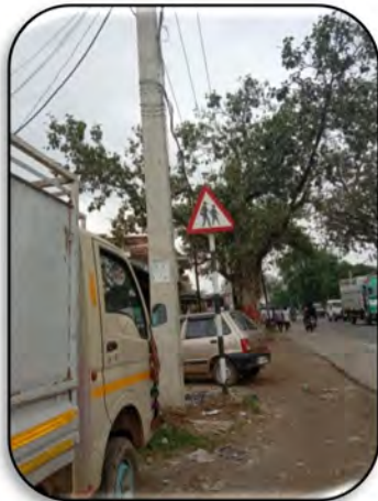
Fig. 6.20: The signage is inappropriately placed
