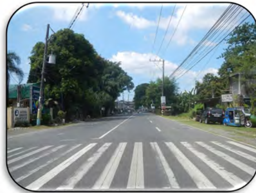
Fig. 6.47: Zebra crossing at NH
