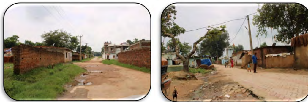
Fig. 6.12: PCC roads which needs maintenance Fig. 6.13: Paved road in the GP
