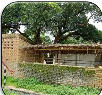
Fig. 4.26: Houses in Neori GP with temporary roof material
