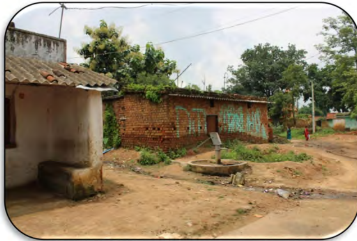
Fig.4.22: Dilapidated house in Neori GP, Source: Author
