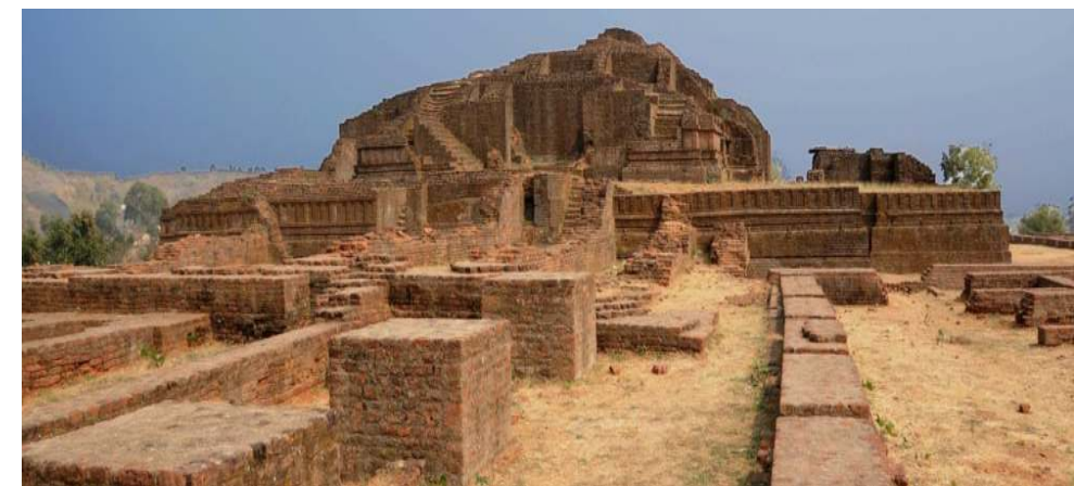
Excavated Brick Structure (A.S.I site) (Source: IncredibleIndia.org.in)
