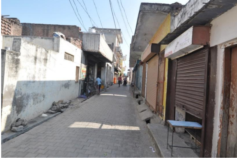
Figure 32: Photograph showing surface drains and street with paver blocks
