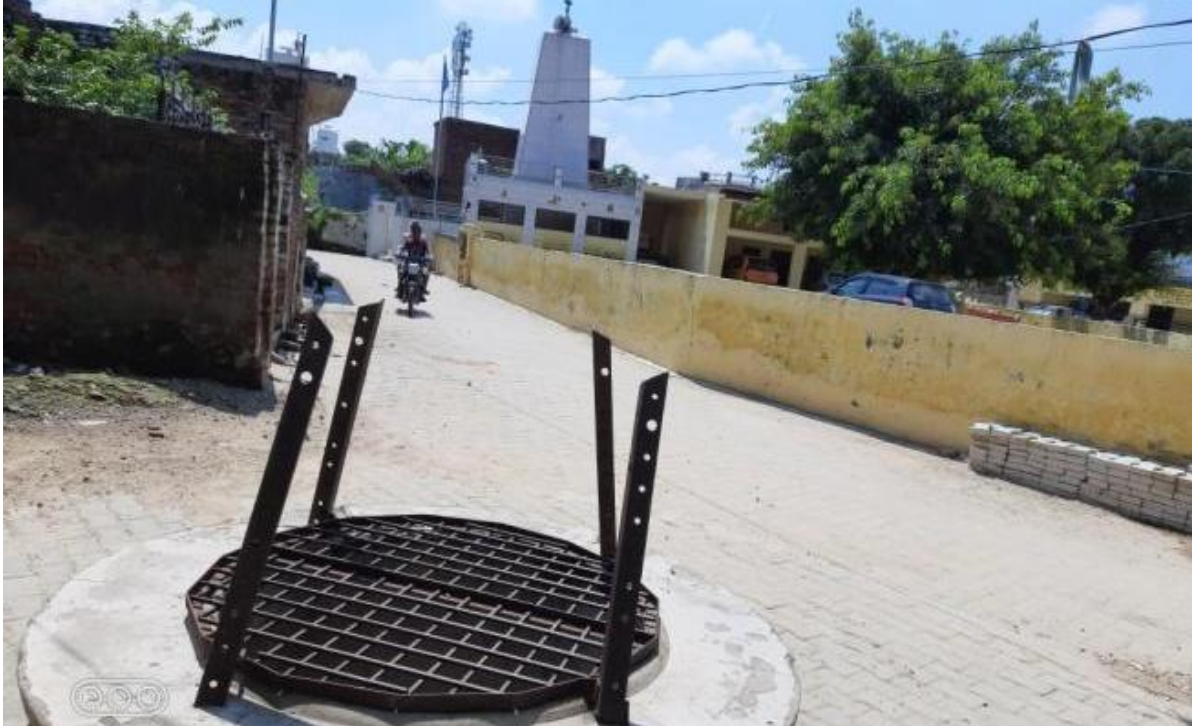
Figure 40: One of the old dry wells in the abadi area
