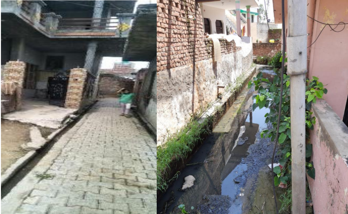
Figure 44: Existing drains and their condition within abadi area
