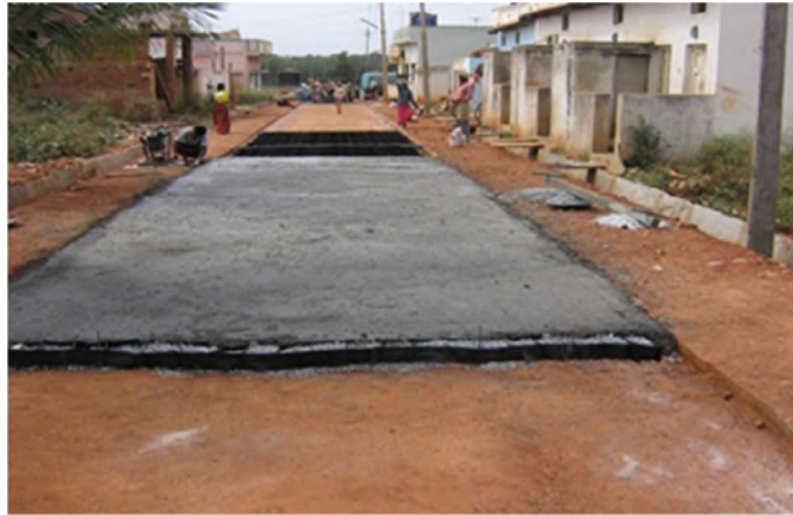
Figure 24: A typical image of cell-filled concrete road for rural areas
