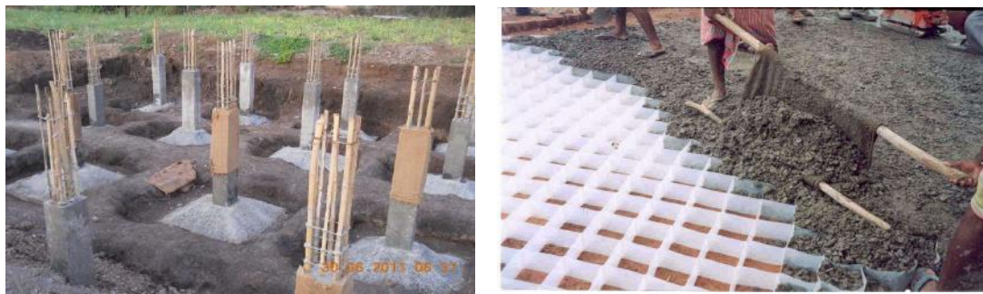
Figure 32: Bamboo-reinforced concrete building technology, and cell-filled concrete technology developed by IIT Kharagpur (which could be adopted at Aguibani GP)
