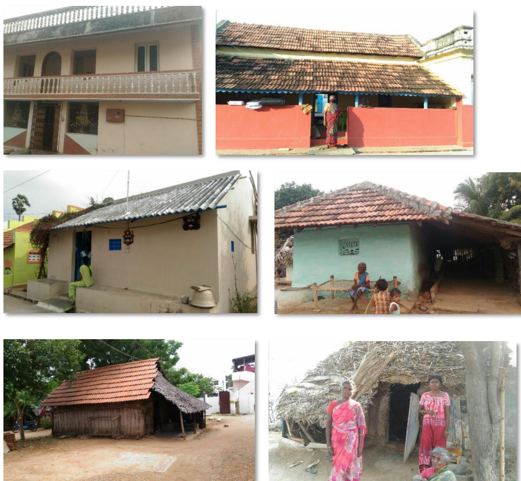
Figure 5.4 Different House Types & construction materials
