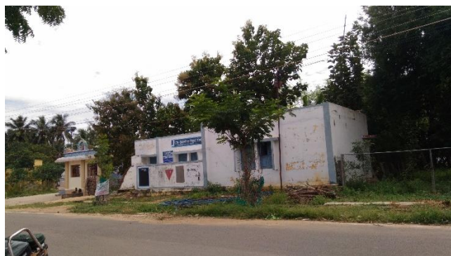
Figure 6.19a: Primary Health Sub centre
