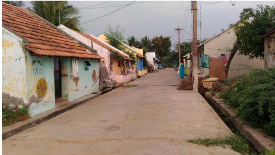
Figure 6.8: Drains on Either side of Streets
