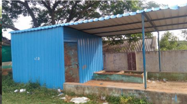
Figure 6.4b: Waste segregation shed
