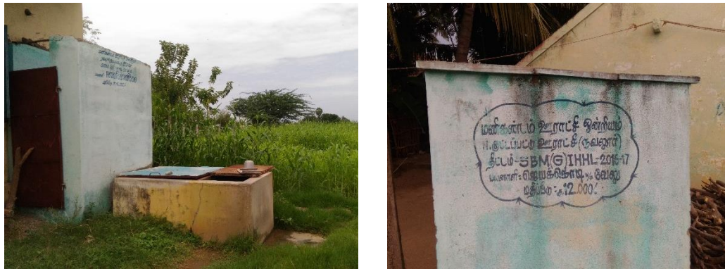
Figure 6.6b: Individual Toilets (Govt. Scheme)
