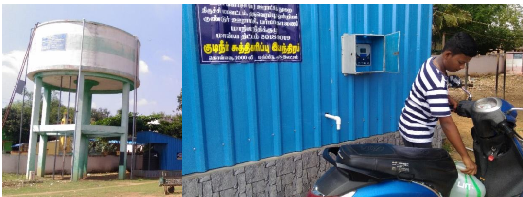
Overhead Water tank
