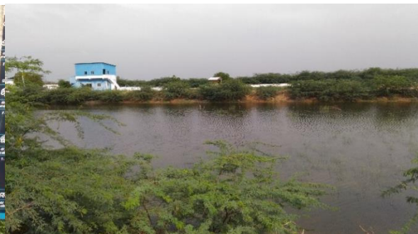
Tannery effluent treatment plant adjacent to Chetti udappu kulam
