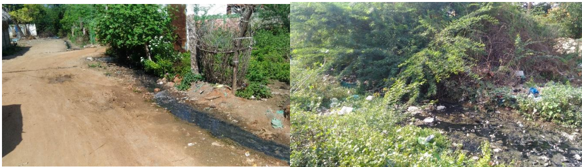
Figure 6.7e: Absence of proper storm water drains and grey water treatment
