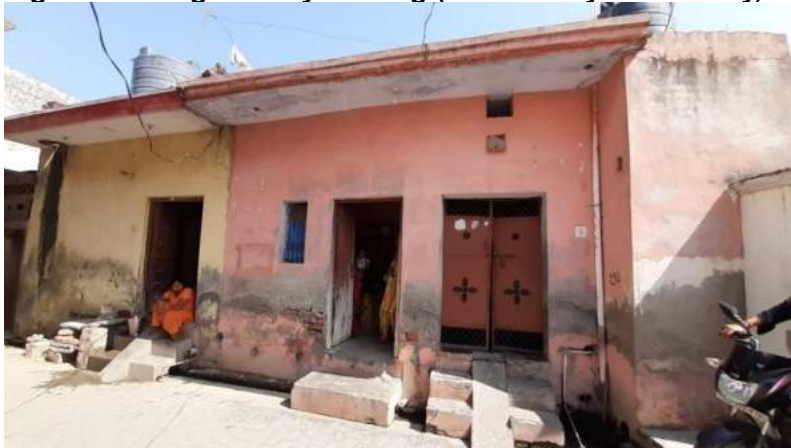
Figure : 65 Single storey building (Source: Physical Survey, Nov 2020)
