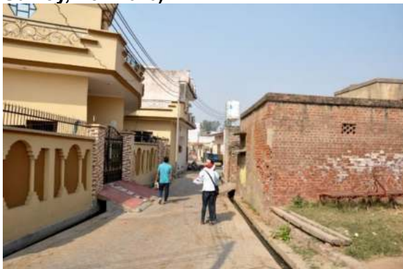
Figure 42 Photograph showing surface drains and street with paver blocks (Source: Physical Survey, Nov 2020)
