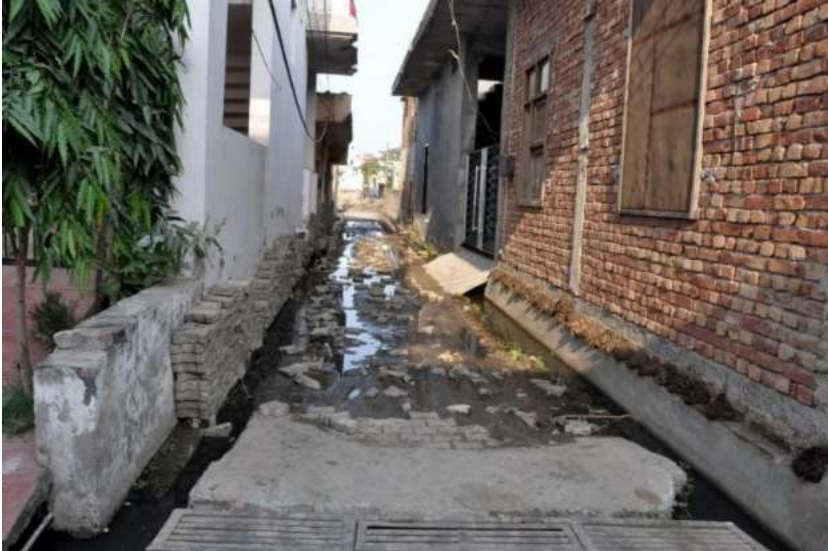
Figure 52 Sewerage pipes opening in street drains (Source: Physical Survey, Nov 2020)
