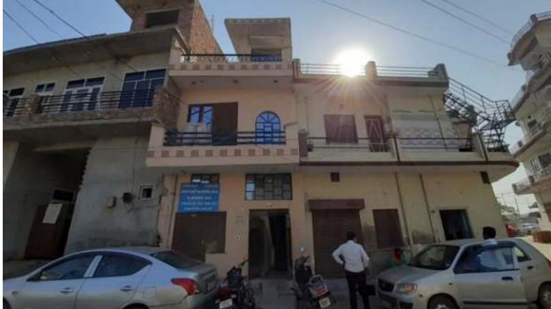
Figure 69 : Double storey Pucca Building (Source: Physical Survey, Nov 2020)
