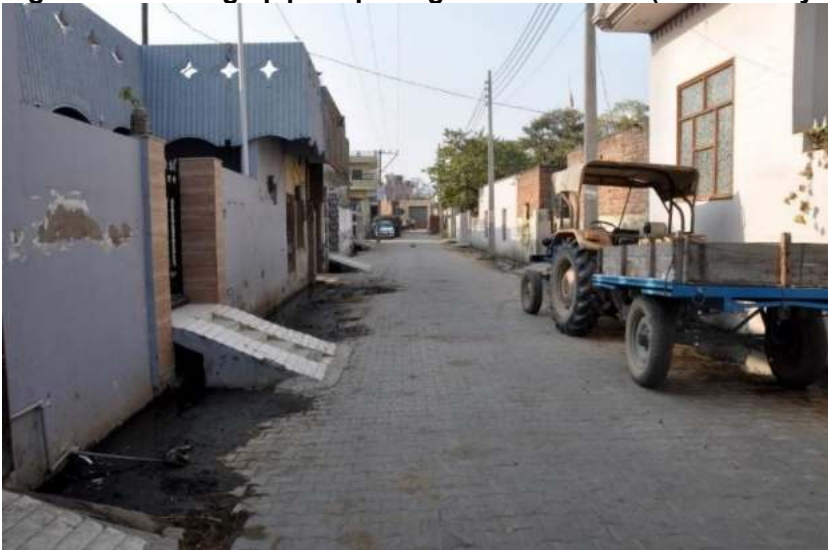
Figure 53 Sewerage pipes opening in street drains (Source: Physical Survey, Nov 2020)
