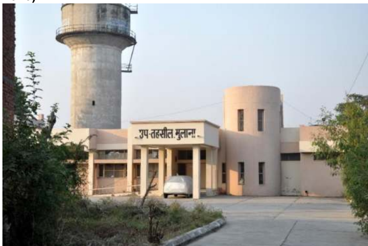
Figure 50 Overhead water tank near Sub Tehsil Office Mullana (Source: Physical Survey, Nov 2020)
