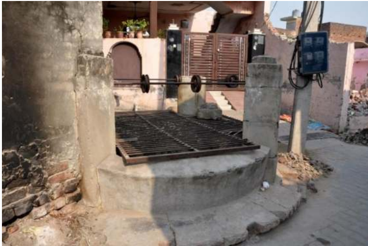
Figure 45 Tubewell connected with underground water tank (Source: Physical Survey, Nov 2020)
