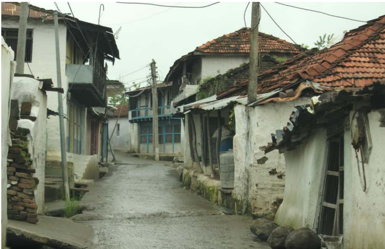
Figure 43 Kuccha houses in oldest settlement of Bilkisganj.
