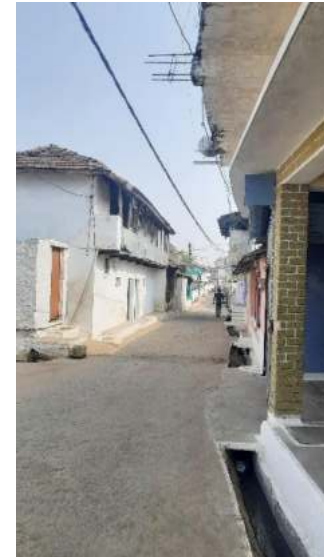
Figure 65 Open drain on one side.
