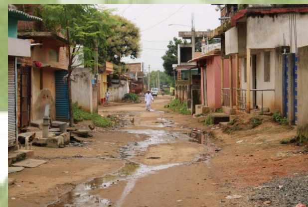
Absence of drainage in almost entire Neori GP
