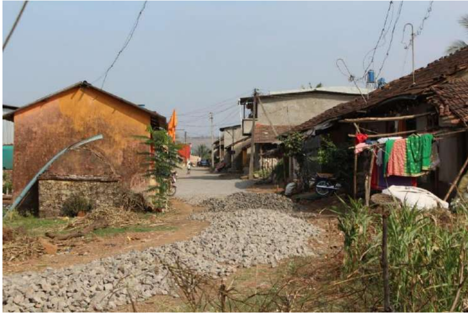
Img 7.3: Ongoing construction and widening of roads
