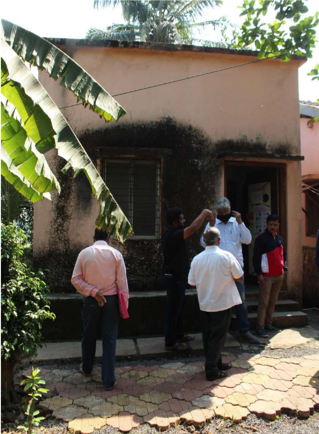
Image 4.2: Bad Condition of Room for Childbirth (Source- Author)
