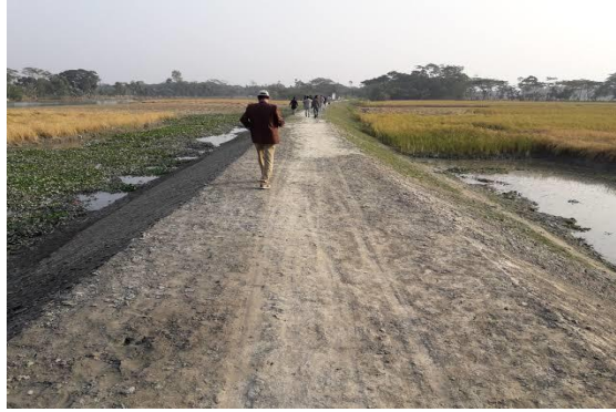
Fig 2.22: Embankment cum road
