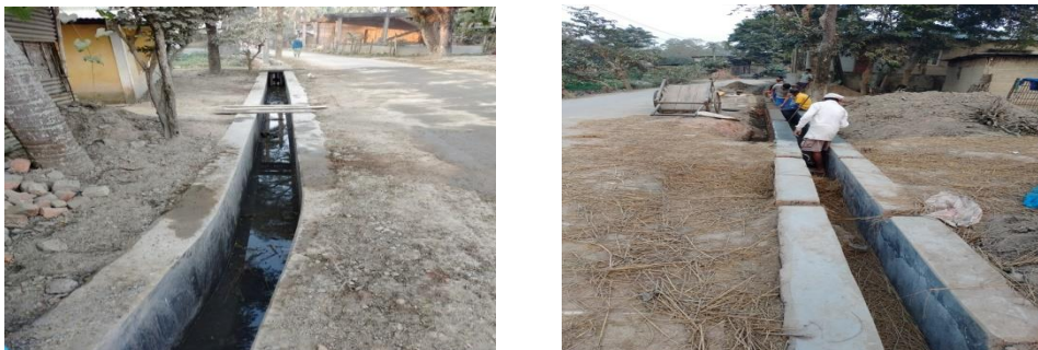
Fig 2.20 Drainage line under construction
