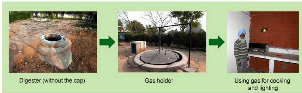
Fig 2.52: Batch-AD system using rice straw and cow dung
