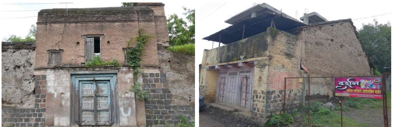
Figure 3:11. Other historic buildings in Belh. Constructed with brick and stone masonry, have fallen in disrepair
