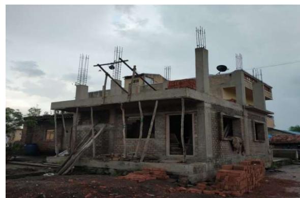
Figure 3:6. Old brick structure and a new RCC Framed structure being constructed in Belhe
