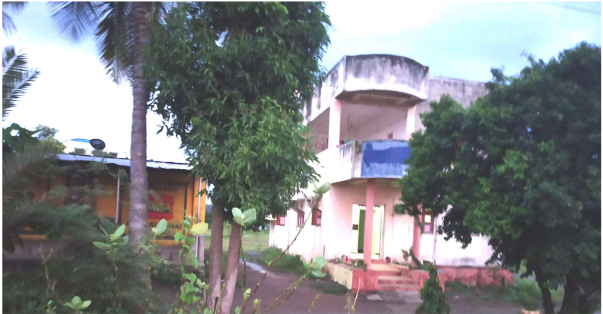
Figure 3:21. Photo of the primary health clinic in Belhe
