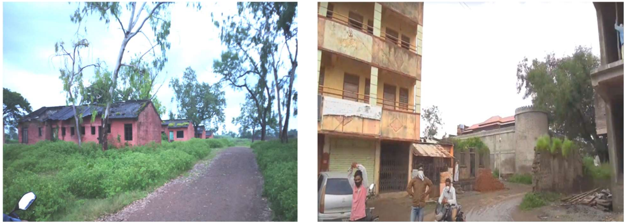
Figure 3.8. Housing at Kukadi colony and other multilevel building
