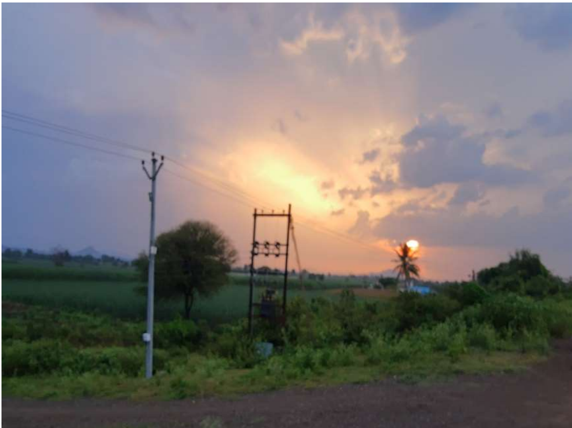
Figure 2:9. Power supply line and pole transformer in Belhe
