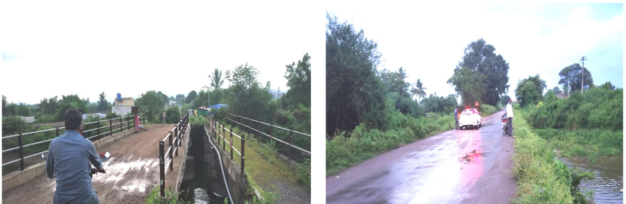
Figure 2:6. Bridge on culvert and further connecting road to the settlement
