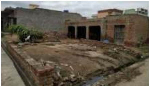
Image 24 Waste dumped st the open drains
