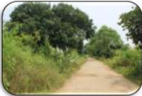
Fig. 7.12: Road (bituminous) which connects Labudih village to NH 32
