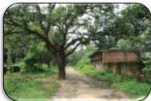
Fig. 7.20: Internal roads are weathered out
