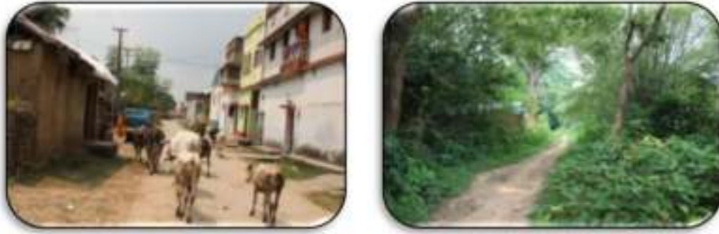
Fig. 7.26: Internal paved roads, Fig. 7.27: Kachha Road at Partanr Partanr from NH 32
