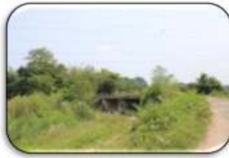
Fig. 7.17: Road (bituminous) which
