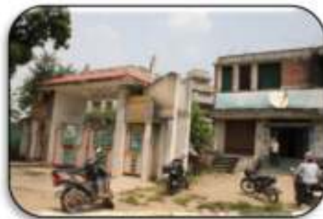
Fig. 7.39: Unorganized parking done in front of the bank.
