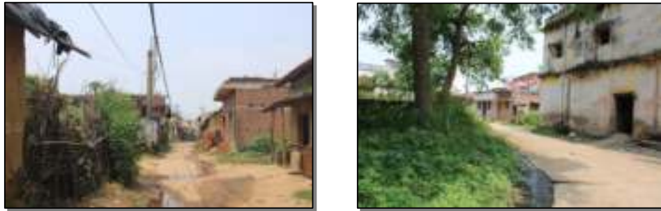
Fig. 6.10: Existing condition of drainage in Kandra GP
