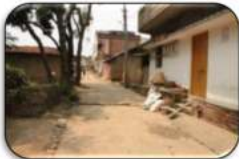
Fig. 7.16: Internal roads (PCC roads)
