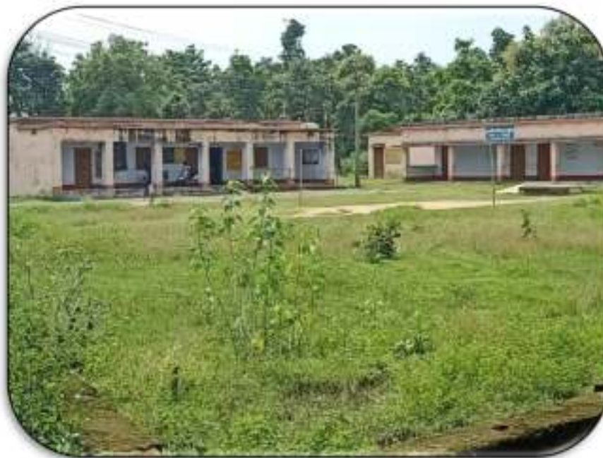
Fig. 4.1: Government Primary School in Kandra GP
