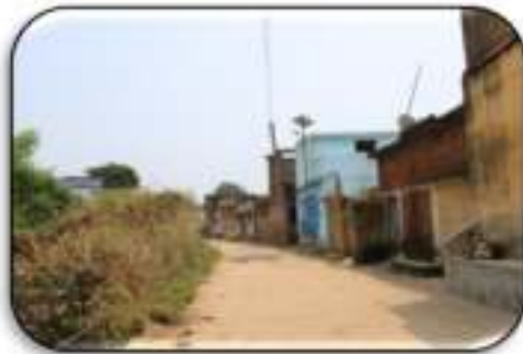
Fig. 7.32: The solar street lights
