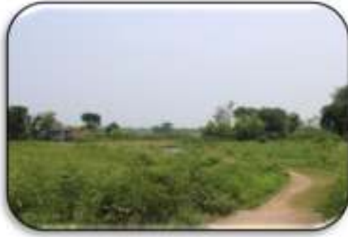
Fig. 7.49: Partially paved road from Kandra to Labudih
