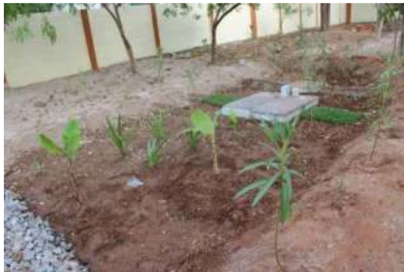
Figure 9-49 Preparation of Soil Bed.
