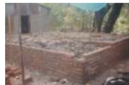
Figure 9-57 Brick plinth construction.
