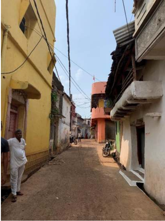
Figure 54 Presence of Open drain on both sides of road within Abadi area.
