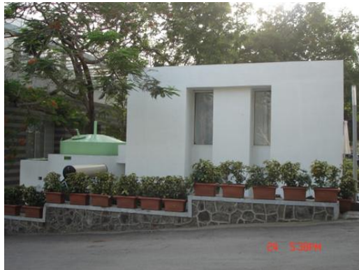
Photo of Nisargruna Biogas plant, TCS, Thane (MS)
