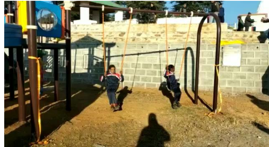
Construction of Parks for children in Pithoragarh by District Panchayat.
