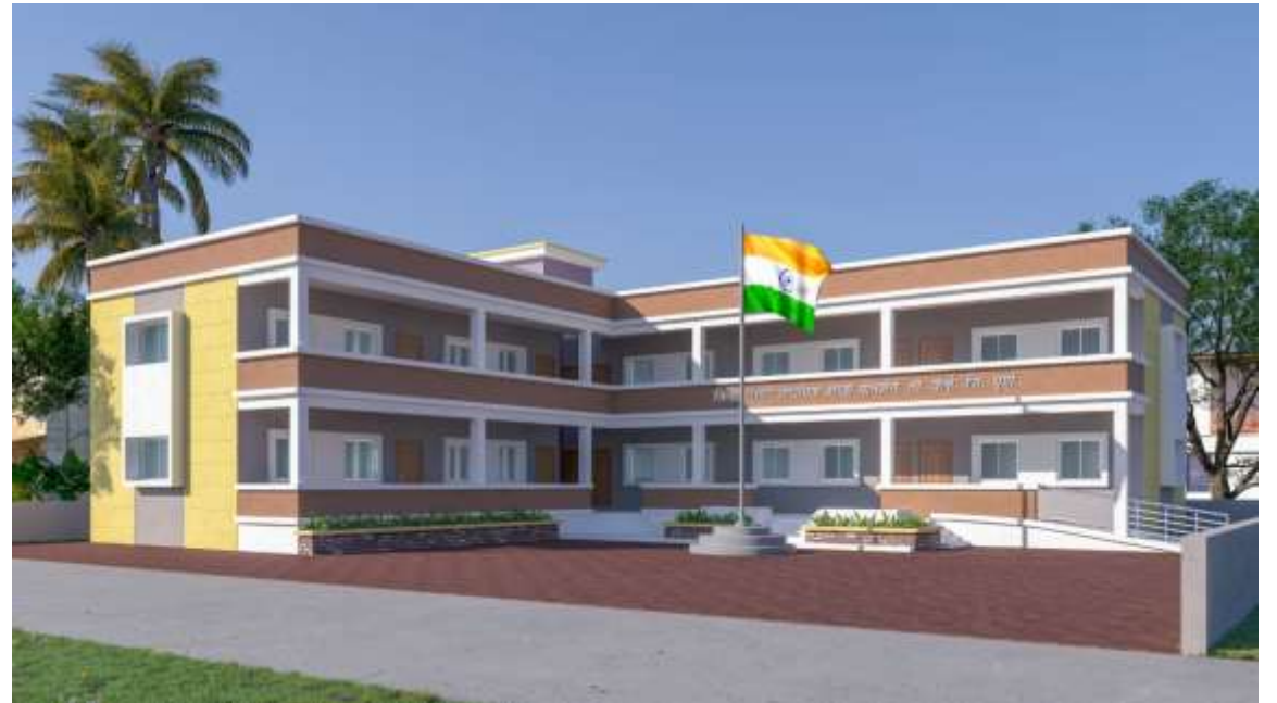
Panshet Cluster School Building
