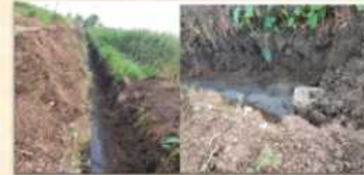
Design and development (in process) of Sewage Treatment Plant
