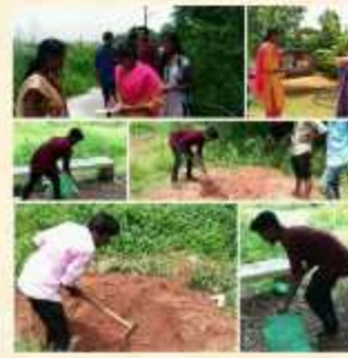
Rain Water Harvesting
