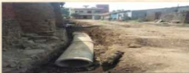
Development of rigid pavement road network and underground drainage system
