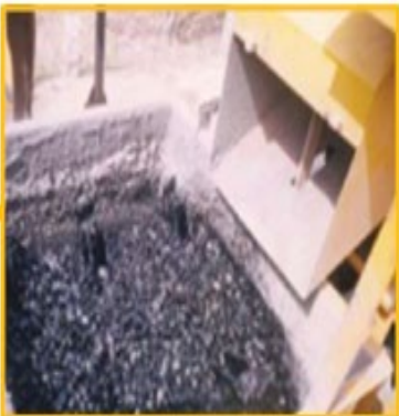
Bitumen added to the coated aggregate
