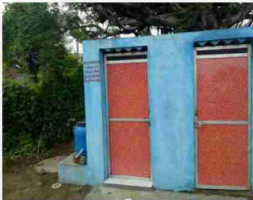
Image: Toilets constructed in the panchayat
