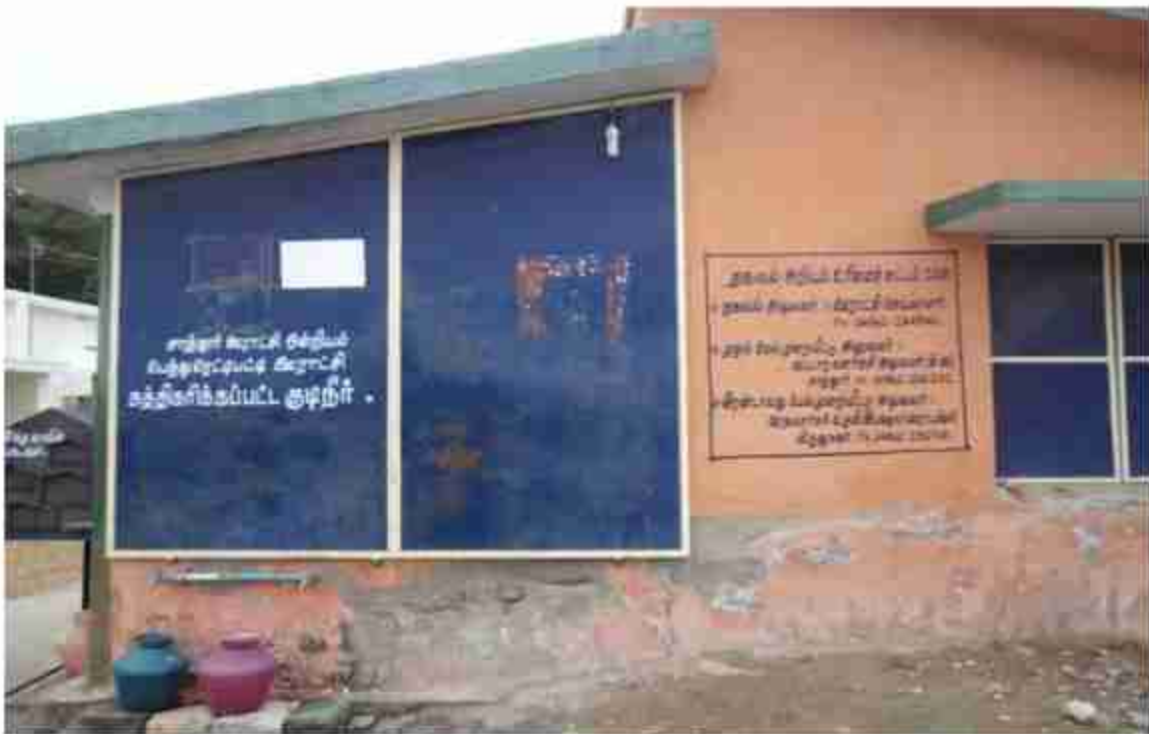
Provision of Potable Water in Pethureddypetty Gram Panchayat
