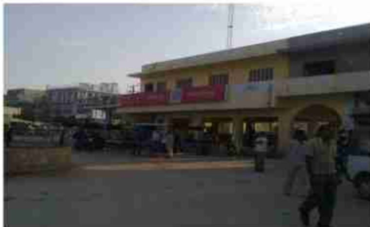
Bank Building, Duni Gram Panchayat, Tonk District
