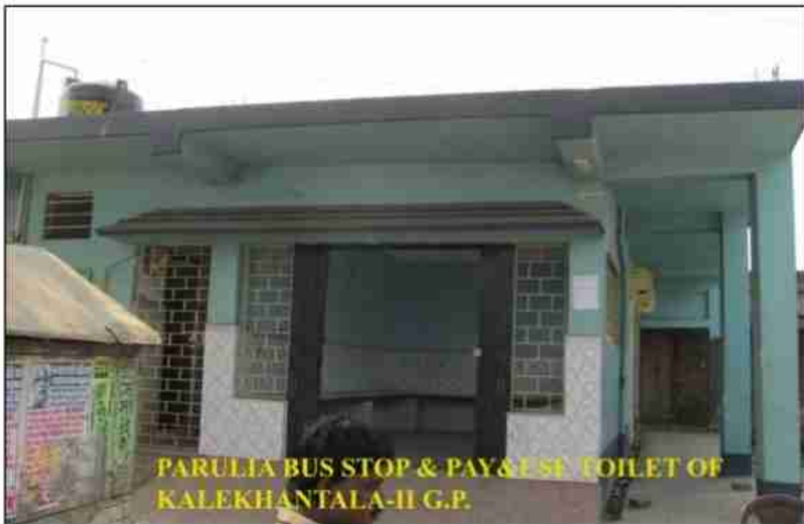
Parulia Bus Stop and Pay and Use Toilet of Kalekhantala – II G.P.
