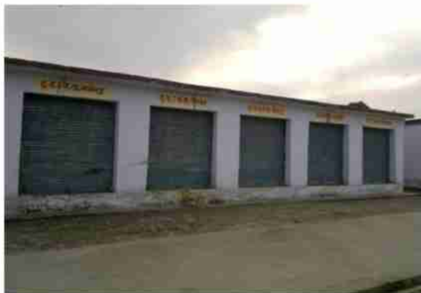
Cemented Roads Constructed in the Market by Balali Gram Panchayat
