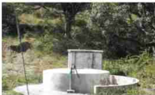
Irrigation Tanks in Hamirpur Pachayat Samiti
