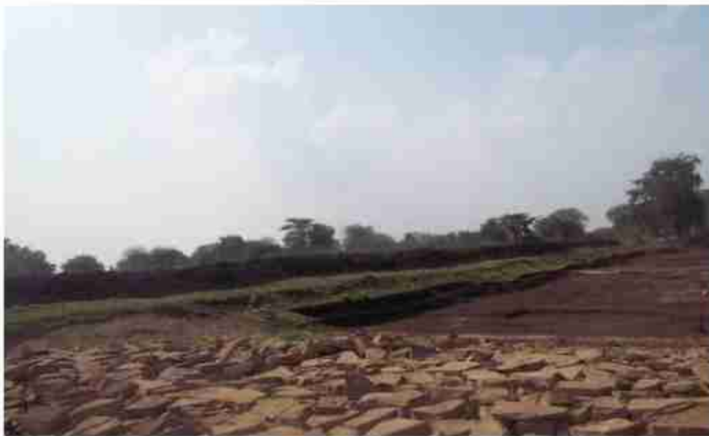
Widening Work of Drain, Daniya Gram Panchayat
