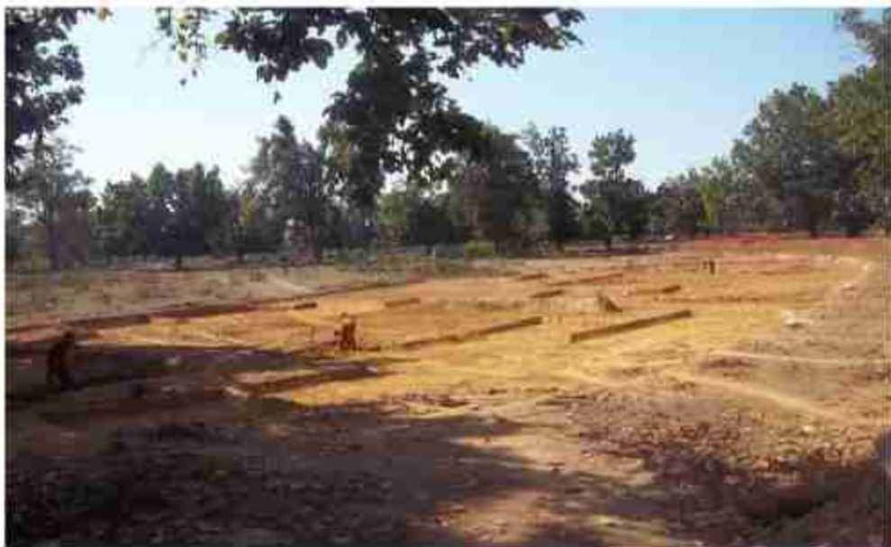
Road Construction under MNREGA in Progress in Amalitikara Gram Panchayat
