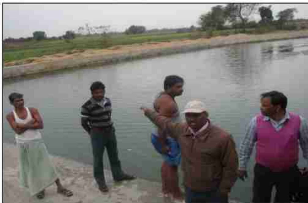
Check Dam constructed by Madhupur Panchayat Samiti
