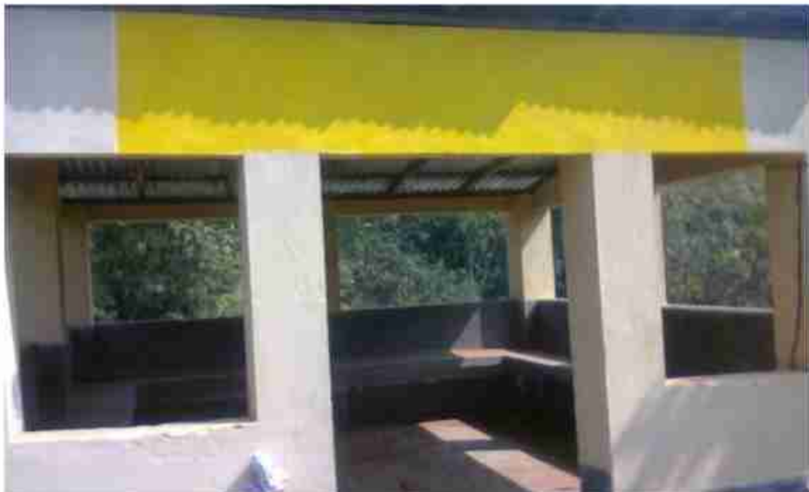
Crematorium Shelter at Amritberia Gram Panchayat
