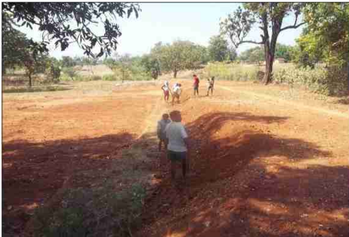
Construction of Link Road under MNREGA Tonahinara Gram Panchayat
