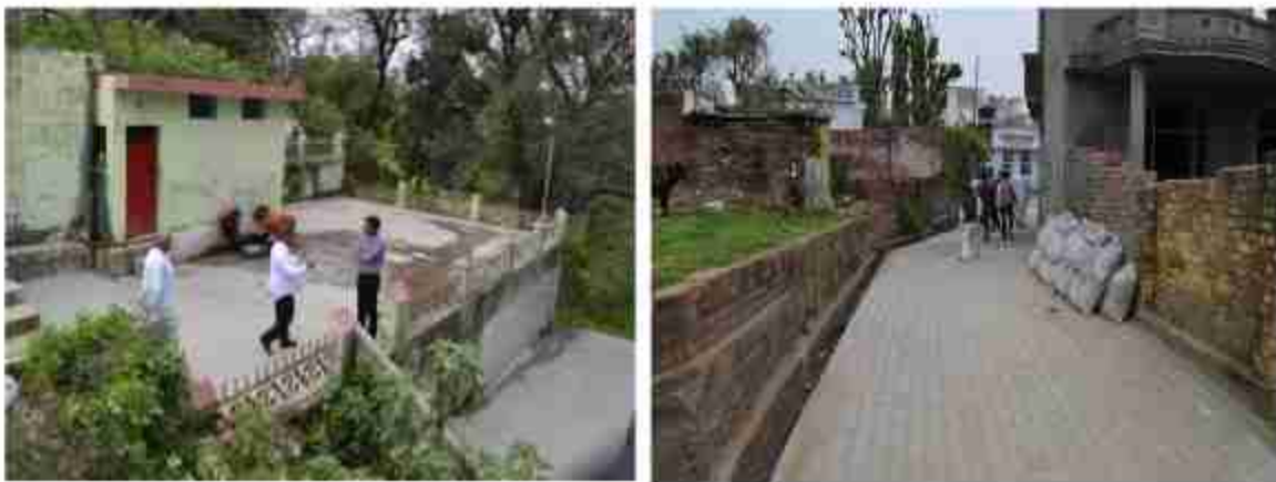
Water Tank, Community Bath and Road Constructed by Kootah Gram Panchayat
