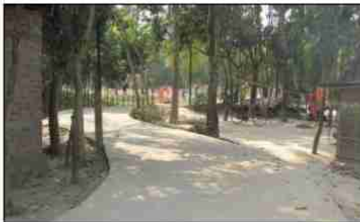
Concrete Road of Kelekhantala – II G.P.
