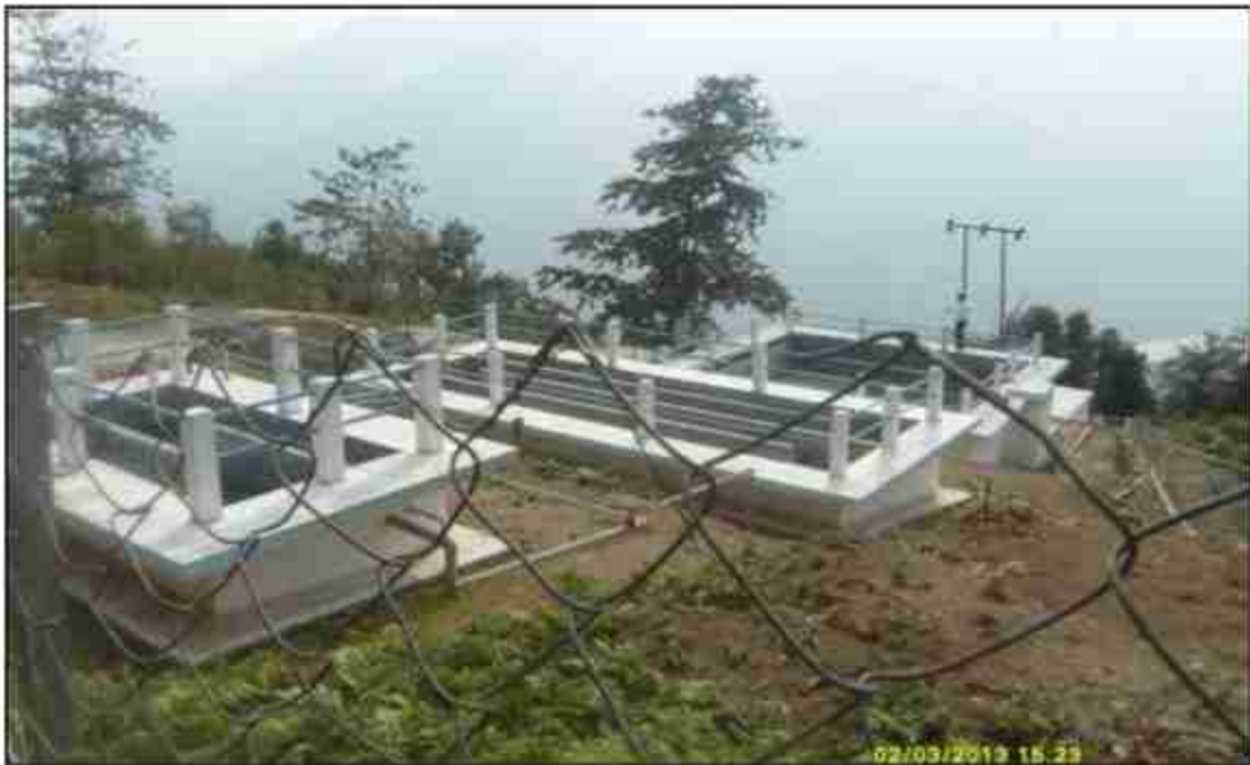
Water Treatment Plant at Simong (West-1) Village
