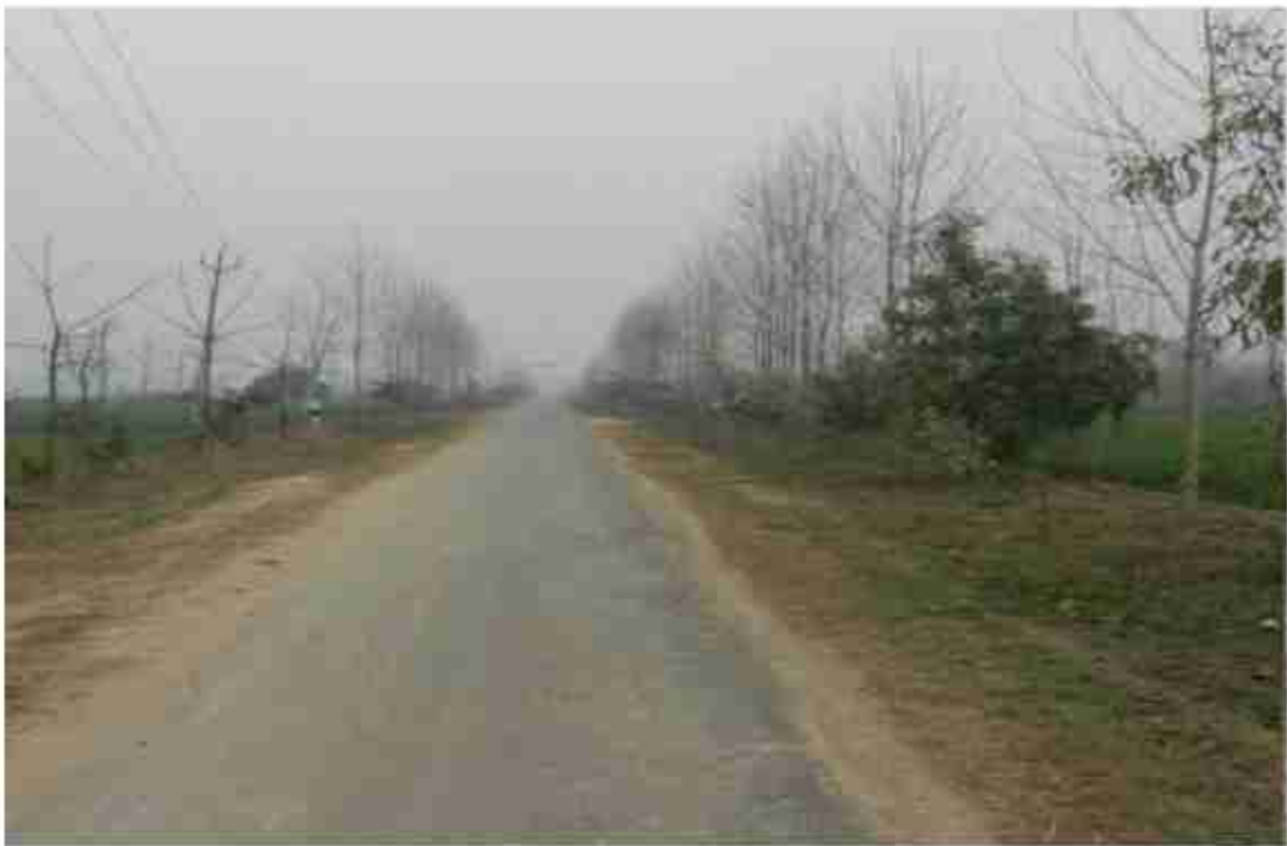
Finished Road with Saplings in Naushera Gram Panchayat
