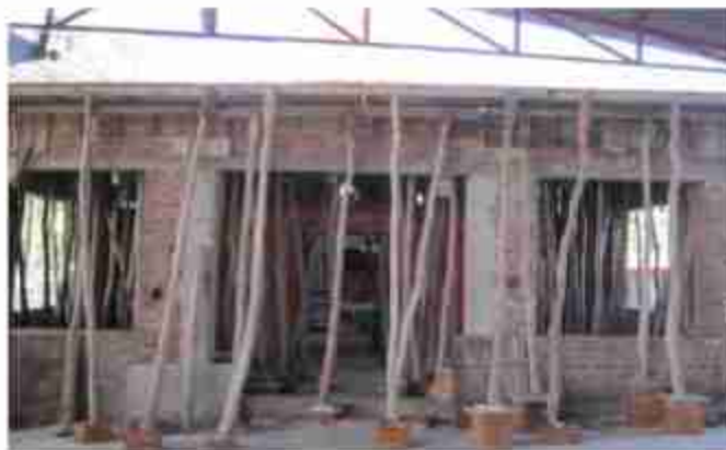
Construction of Room for Tourists in Javla Gram Panchayat
