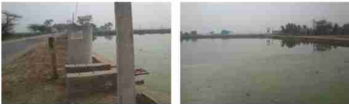
Construction of Boundary Around the Pond by Hukumsinghwala Gram Panchayat
