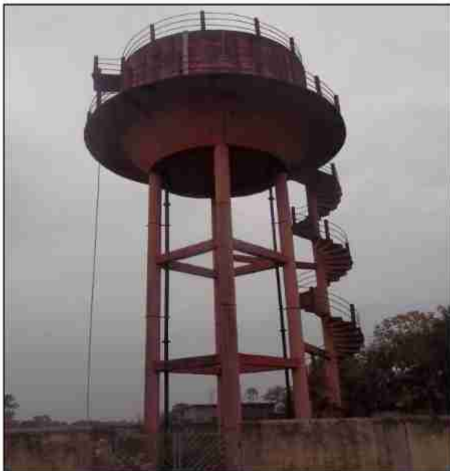
Water Tank built by Jhalmala Gram Panchayat
