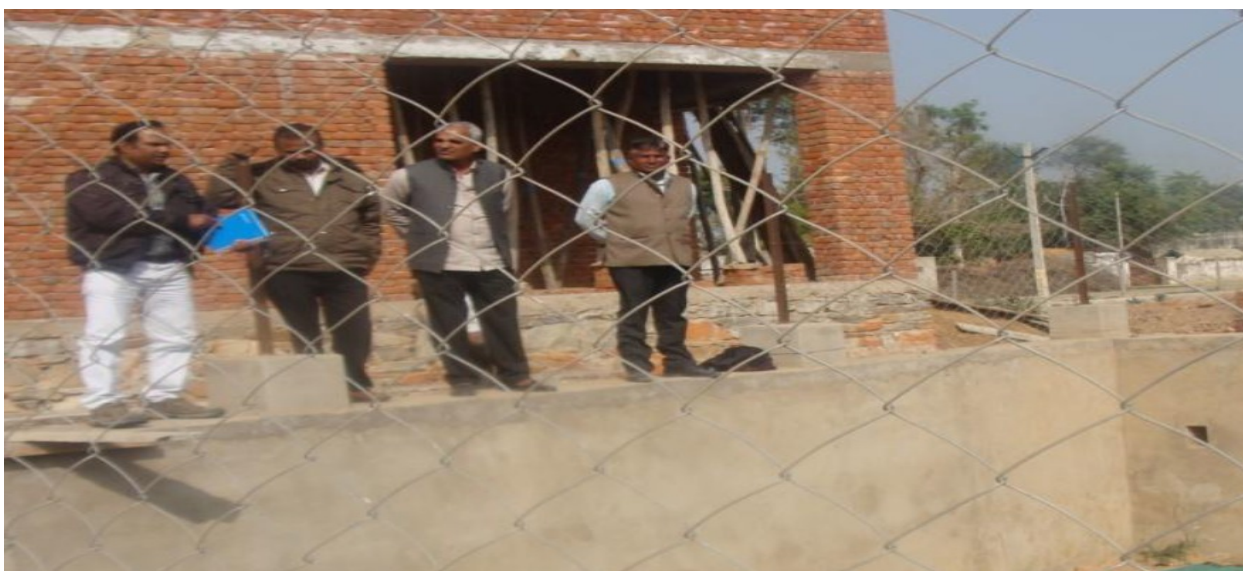
Picture of Construction of Water Recharge Well
