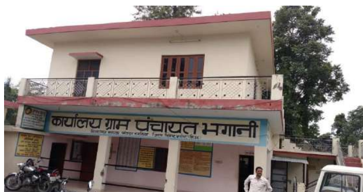
Construction of Gram Panchayat Building under BRGF in Bhangani GP, Sirmaur District, Himachal Pradesh State
