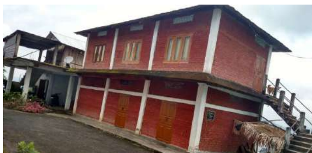
Construction of community hall under BRGF at Goching Village, Mon District, Nagaland State
