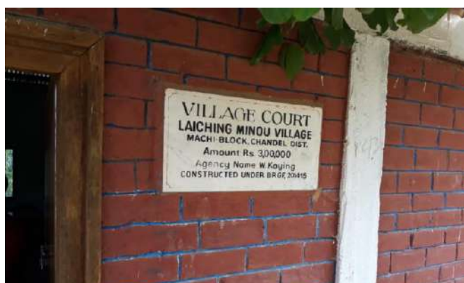
Building for Village Court constructed under BRGF Laiching Minou Village, Machi Block in Chandel district, Manipur State
