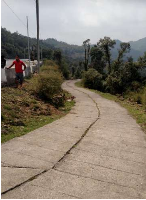
Construction of link road under BRGF in Dilman GP, Sirmaur District, Himachal Pradesh State
