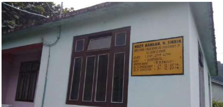
Construction of PHC Quarters under BRGF Passing Saffo GP, Passing Dzongu Block, North Sikkim, Sikkim State
