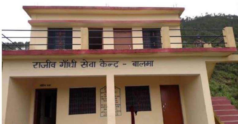
Construction of Rajiv Gandhi Seva Kendra under BRGF in Bamla GP. Tehri Garhwal District. Uttarakhand State
