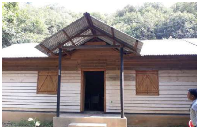
Construction of Residential Hostel under BRGF (Leishokching Village, Chandel Block, Chandel District)-
