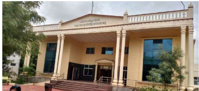
Construction of Kuvembu Cultural Centre under convergence with BRGF in Davangere Municipal Corporation, Davangere District, Karnataka State
