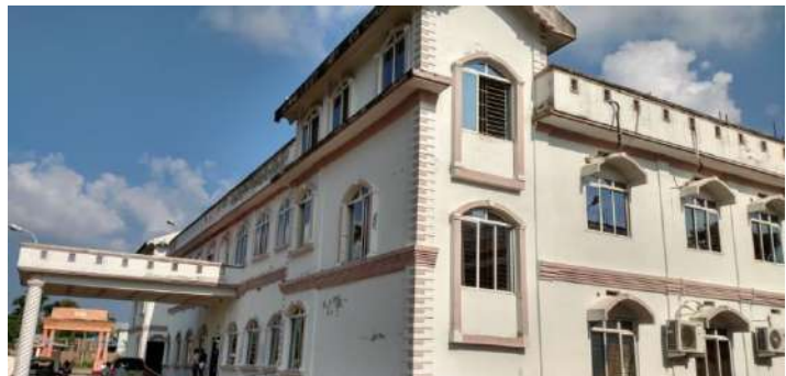
Construction of Building under BRGF for PRTI- Lalchari in Ambassa Municipality, Dhalai District, Tripura State
