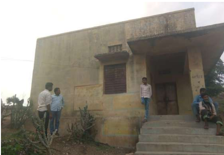
Building for Veterinary Sub Centre constructed under BRGF in Baleecha GP, Girwa Block, Udaipur District, Rajasthan State
