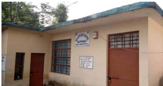
Construction of Health Sub Centre under BRGF in Ambwala Santwala GP, Sirmour District, Himachal Pradesh
