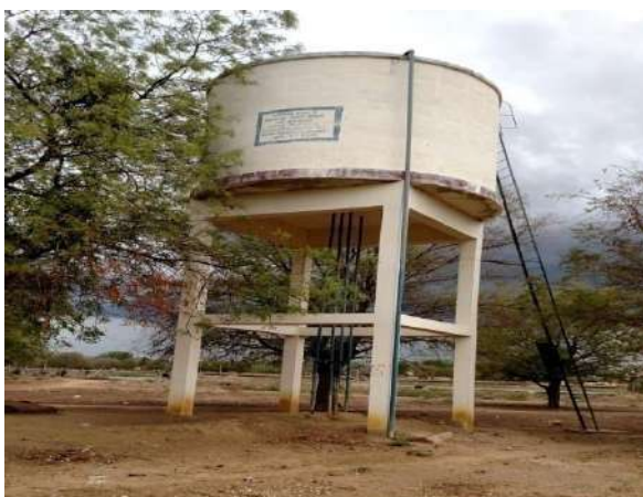
Construction of OHT and Borewell under BRGF in Kandadevi VP, Sivaganga District, Tamil Nadu State
