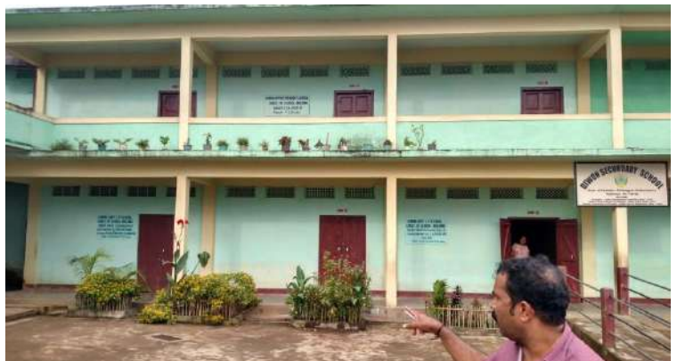
Construction of school building under BRGF in Diwon GP, Umling Block, Ri- Bhoi District, Meghalaya State
