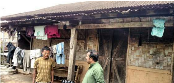
Construction of House under BRGF in Longching GP, Mon District, Nagaland State
