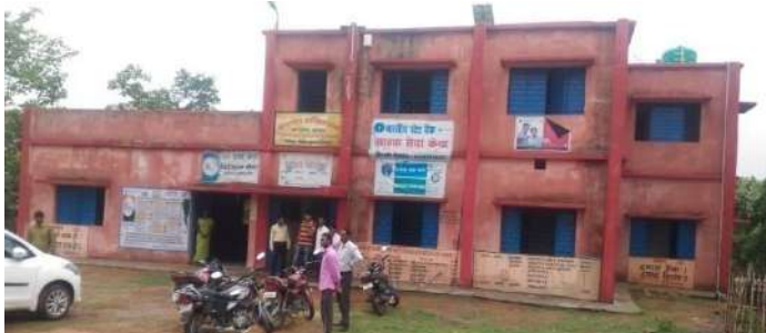
Gram Panchayat Building under BRGF Jai Nagar GP, Ramgarh District, Jharkhand State
