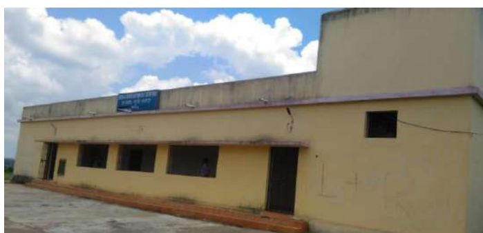
Construction of Skill Development Centre under BRGF at Sunabeda Municipality, Koraput District, Odisha State
