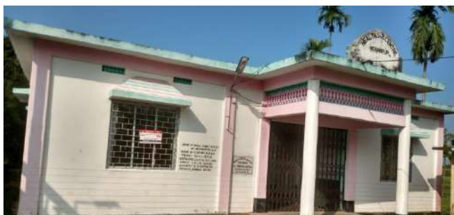
Construction of Health Centre under BRGF in Mohanpur GP, Dhalai District, Tripura State
