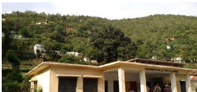
Construction of Rajiv Gandhi Seva Kendra under convergence with BRGF in Chippara GP, Tehri Garhwal District, Uttarakhand State
