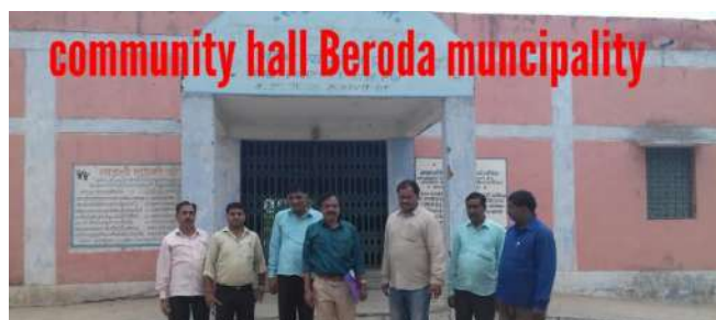
Community hall constructed under BRGF at Baroda Municipality, Sheopur District, Madhya Pradesh
