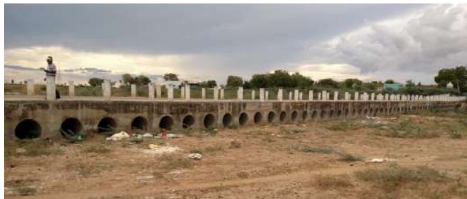
Construction of bridge under BRGF at Virusali river in Thirumanavayal VP, Sivaganga District, Tamil Nadu State
