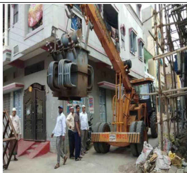
Representative photograph showing crane used in residential area to replace transformer. (Source: The Hans India)
