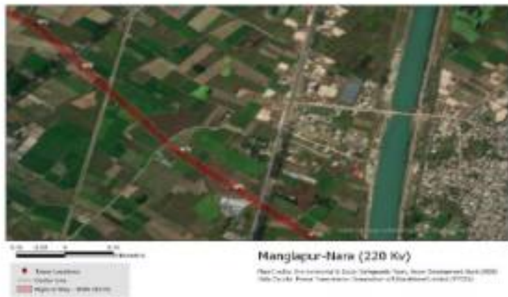
Figure 5. Mangapur-Narva Power Line- View of Polysilicon Tower AC-4 to AC-10
