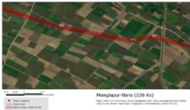
Figure 2: Manglapur-Nara Power Line-View of Right of Way Tower AT-13 to AT-17
