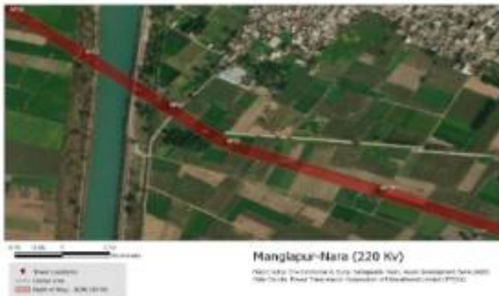
Figure D: Mangapur-Nara Power Line-View of Horizontal Tower AP-11 to AP-14
