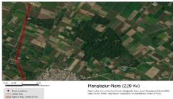
Figure 3: Mangalore-Nam Power Line: View of Mangalore-Nam Power Line 220 Kv to 220 Kv
