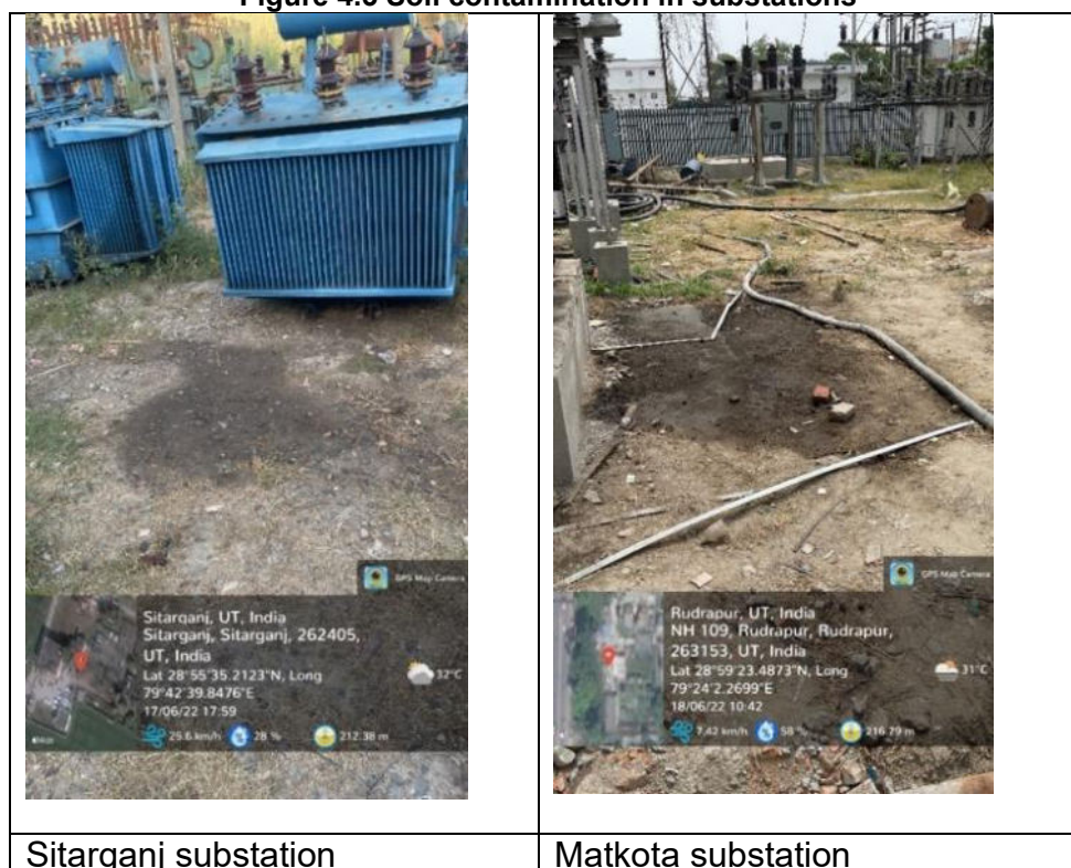
Figure 4.3 Soil contamination in substations
