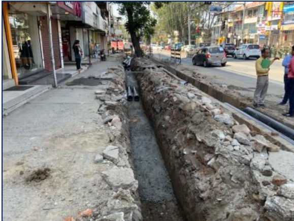
Figure 11: Open Trench with Buried Pipes, Dehradun
