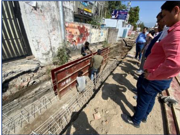
Figure 12: Covered Chamber Construction, Dehradun
