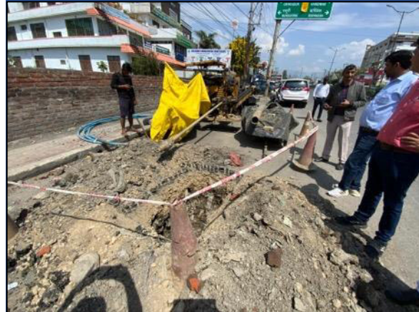
Figure 15: HDD Drilling Machine, Dehradun
