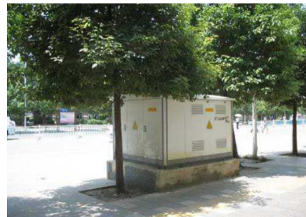
Figure 16: Examples of Compact Substations
