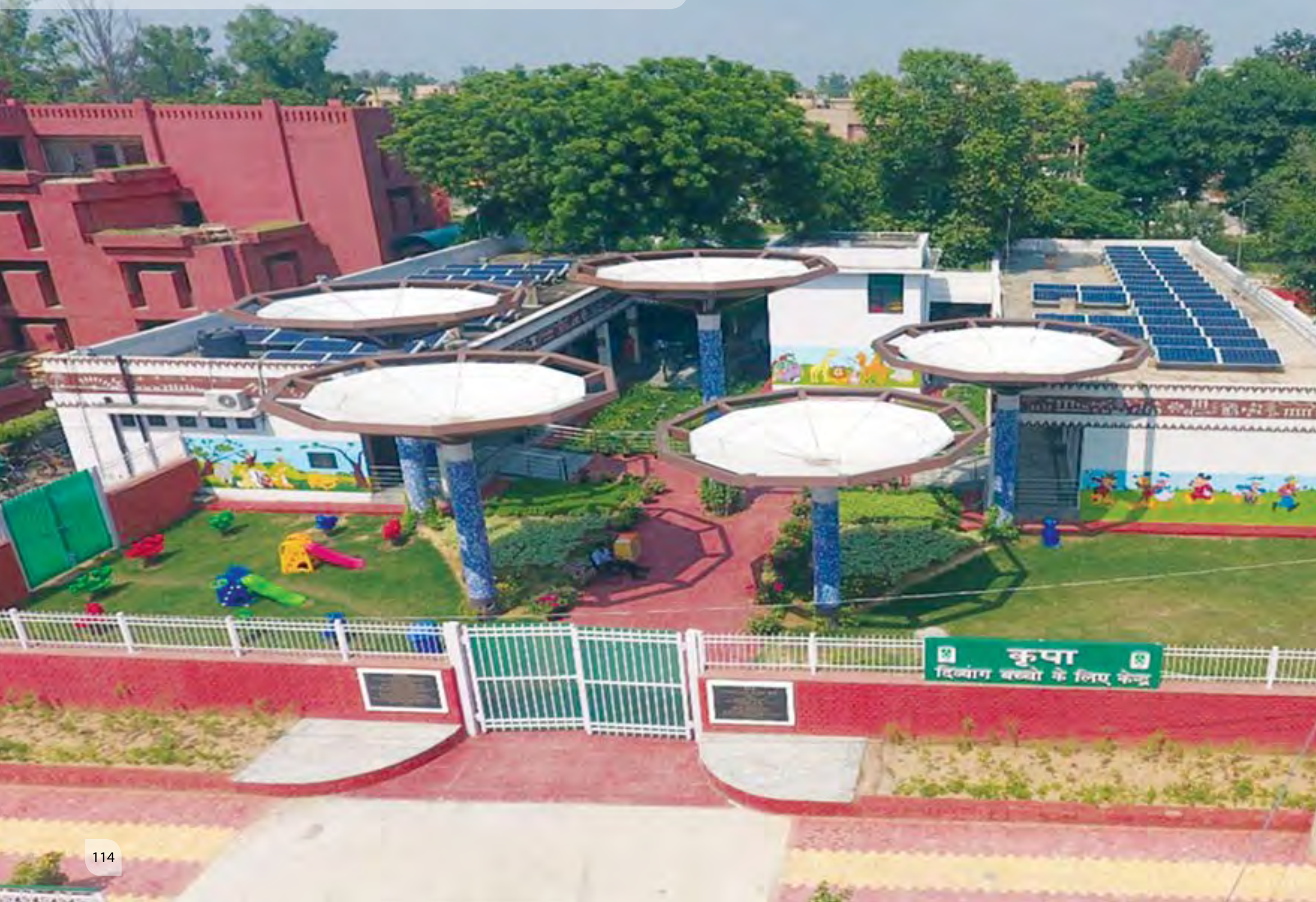
Rain Water Harvesting at Kripa Special School, Delhi Cantonment
