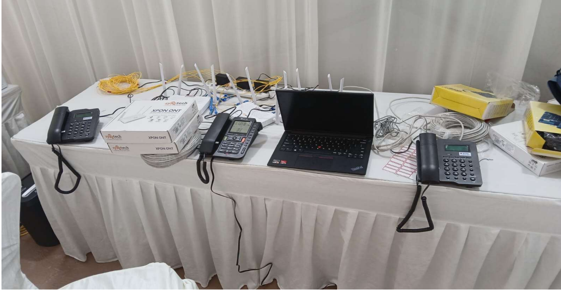
DIO/DIA Kurnool Coordinating the Technical Infrastructure arrangements at the Event
